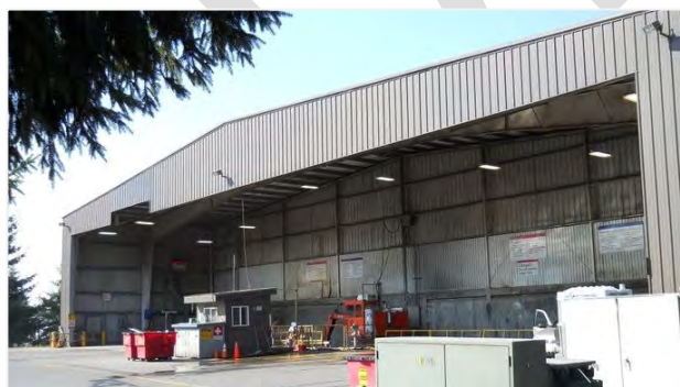
North County Recycling and Transfer Station
