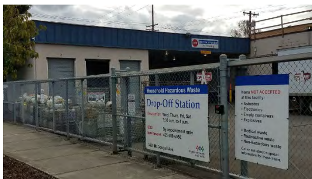
Moderate Risk Waste Facility
