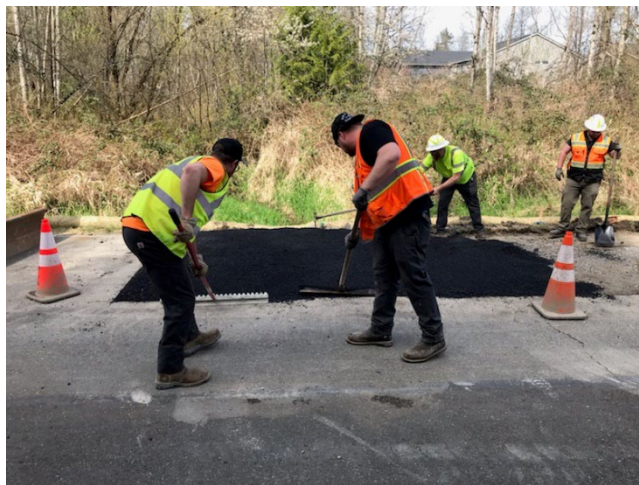
Culvert Repair - 36th Street NE
