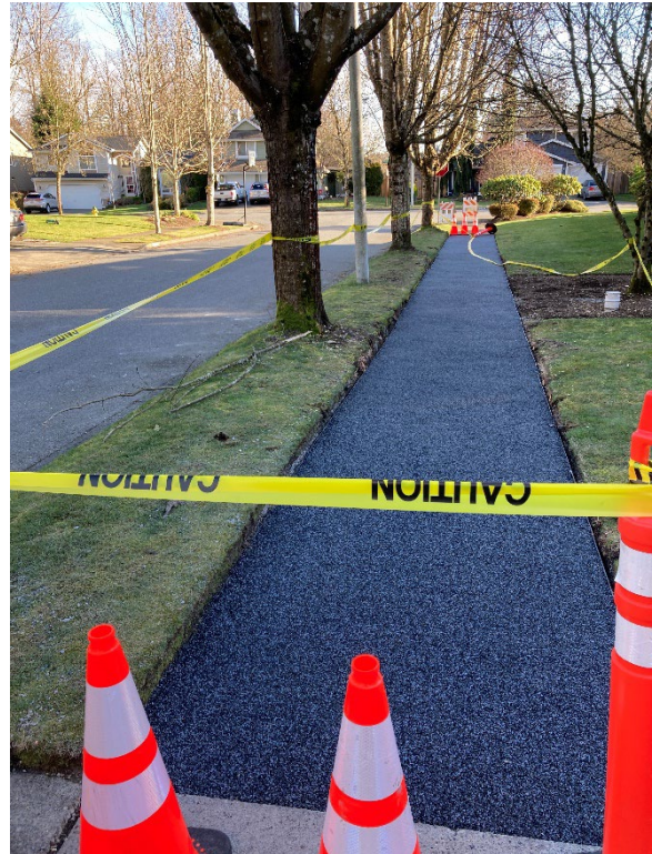
Sidewalk Repair Due to Root Damage, concrete replaced with alternative surface to retain trees. Photo from 2023.
