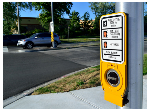
Figure 2-15 “H-style” (above) and APS-style pedestrian pushbutton (below)
