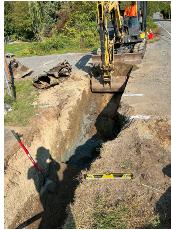
Replacement in Progress
