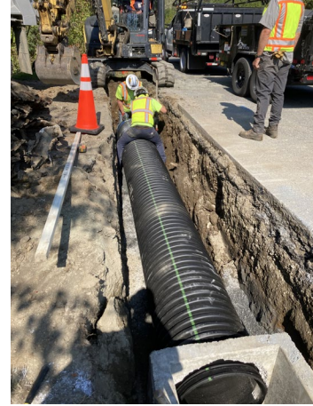
New Pipe Installation
