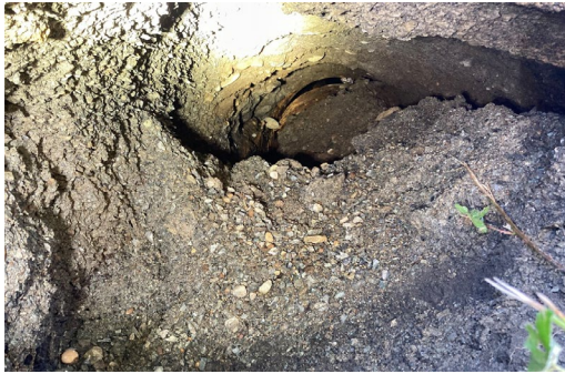
Collapsed Culvert
