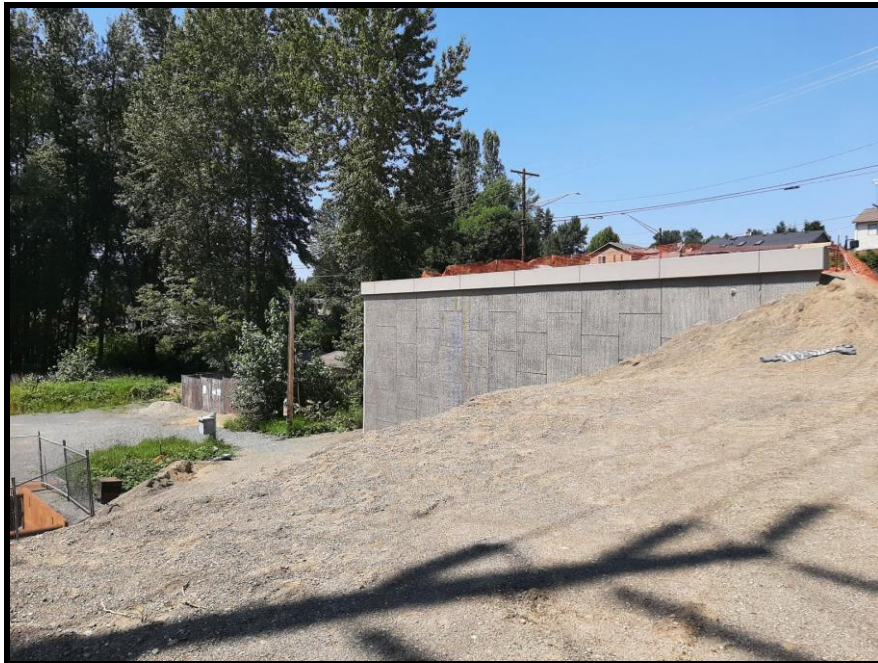
4. View of building structure.
