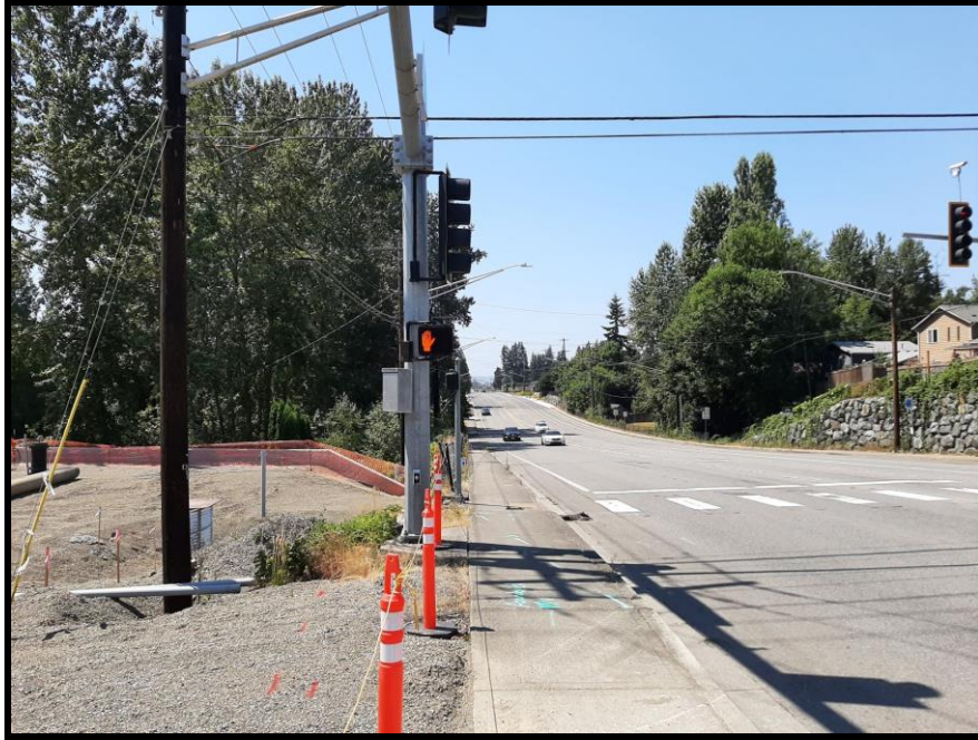
1. Westerly view along 20 th St SE.
