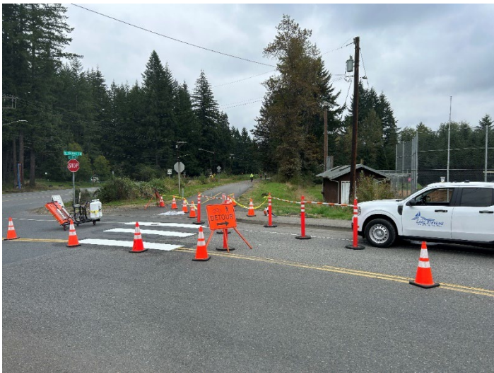
City Crews Installing Thermoplastic on 16th Street NE
