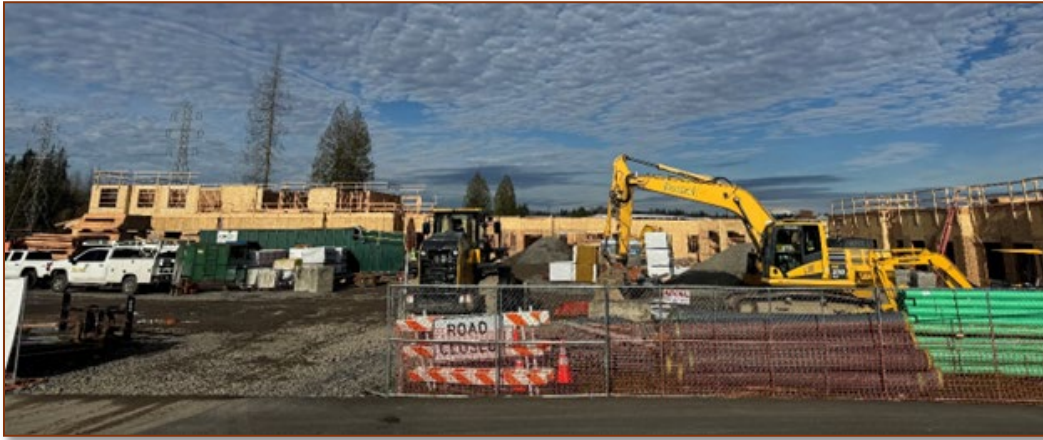
Village Concepts Assisted Living Facility Under Construction
