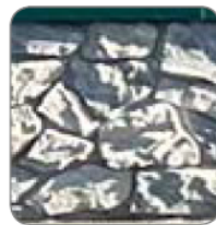
4 Existing Stone Cladding
