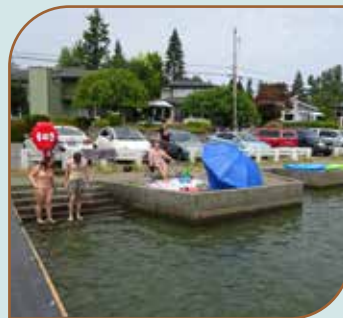
North Lakeshore Beach renovated with new swim dock decking.
