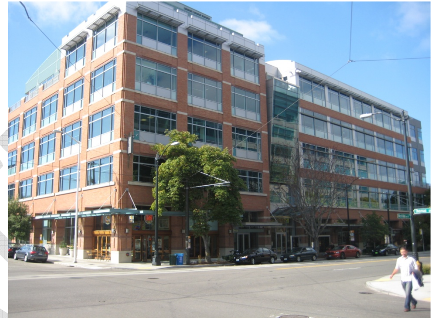
Figure 6.9 Photo of Office over Retail building
